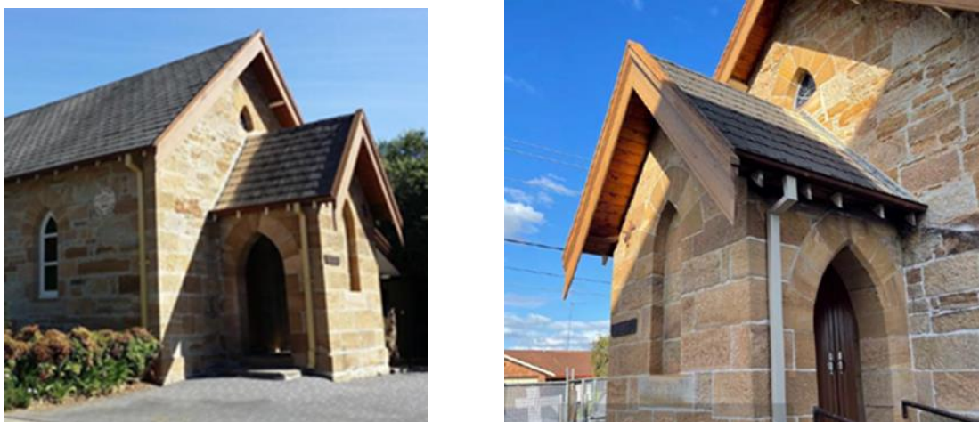
Figure 4: Views of the existing chapel (Source: Group GSA)
