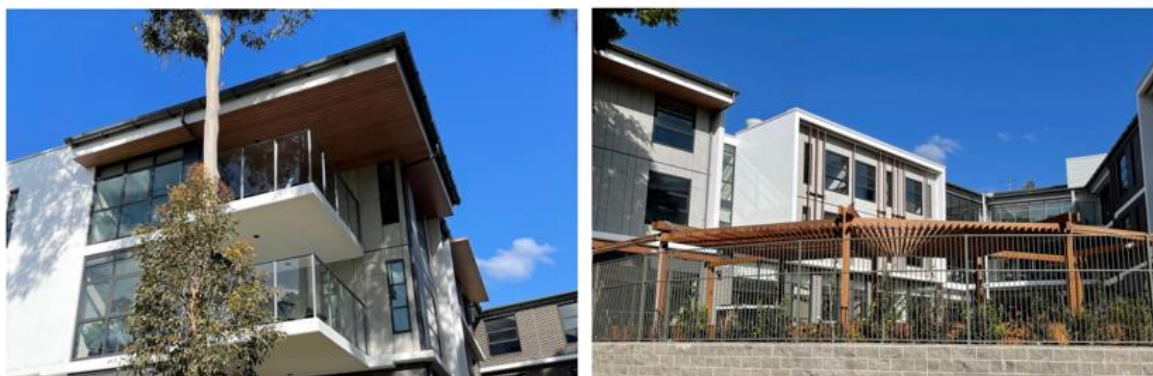
Figure 2: Edinglassie Residential Aged Care Facility - approved under DA 18/0306 (Source: Group GSA)
